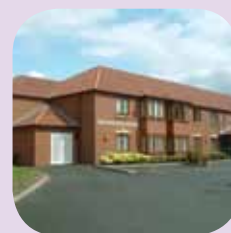
Braeburn House, Walsall
